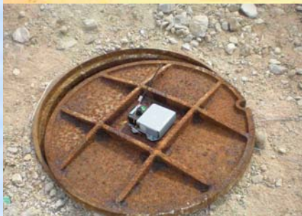
Installed SmartCover Unit Magnetic Mount
